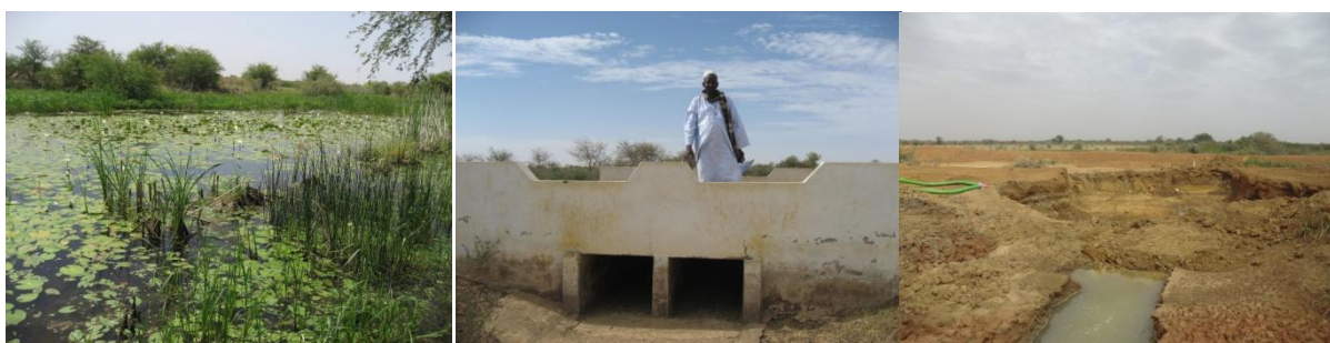
Pont Alain Daniel is a nice and diverse place, when there is water (left picture, e.g. Oct. 2012), and a logical stop during excursions in the Ndiael (middle). It is being removed in February 2015 (right picture) to allow for the passage of larger volumes of water in the near future by PREFELAG. The Yéti Yone is dammed during these works.
