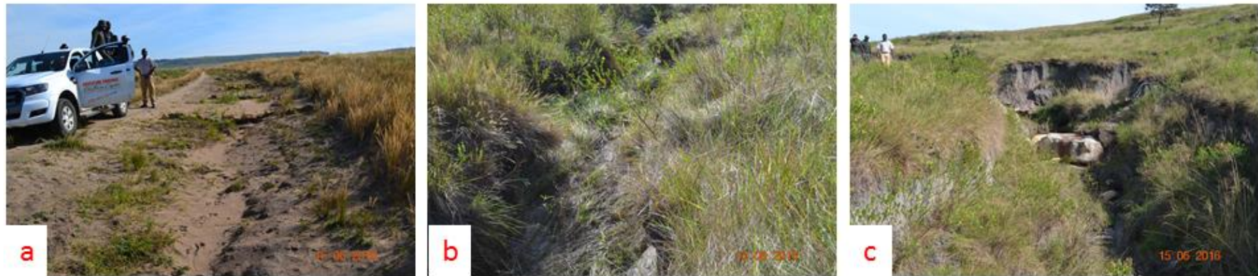
Figure 2. Wetland degradation caused by water runoff from roadside – donga erosion
