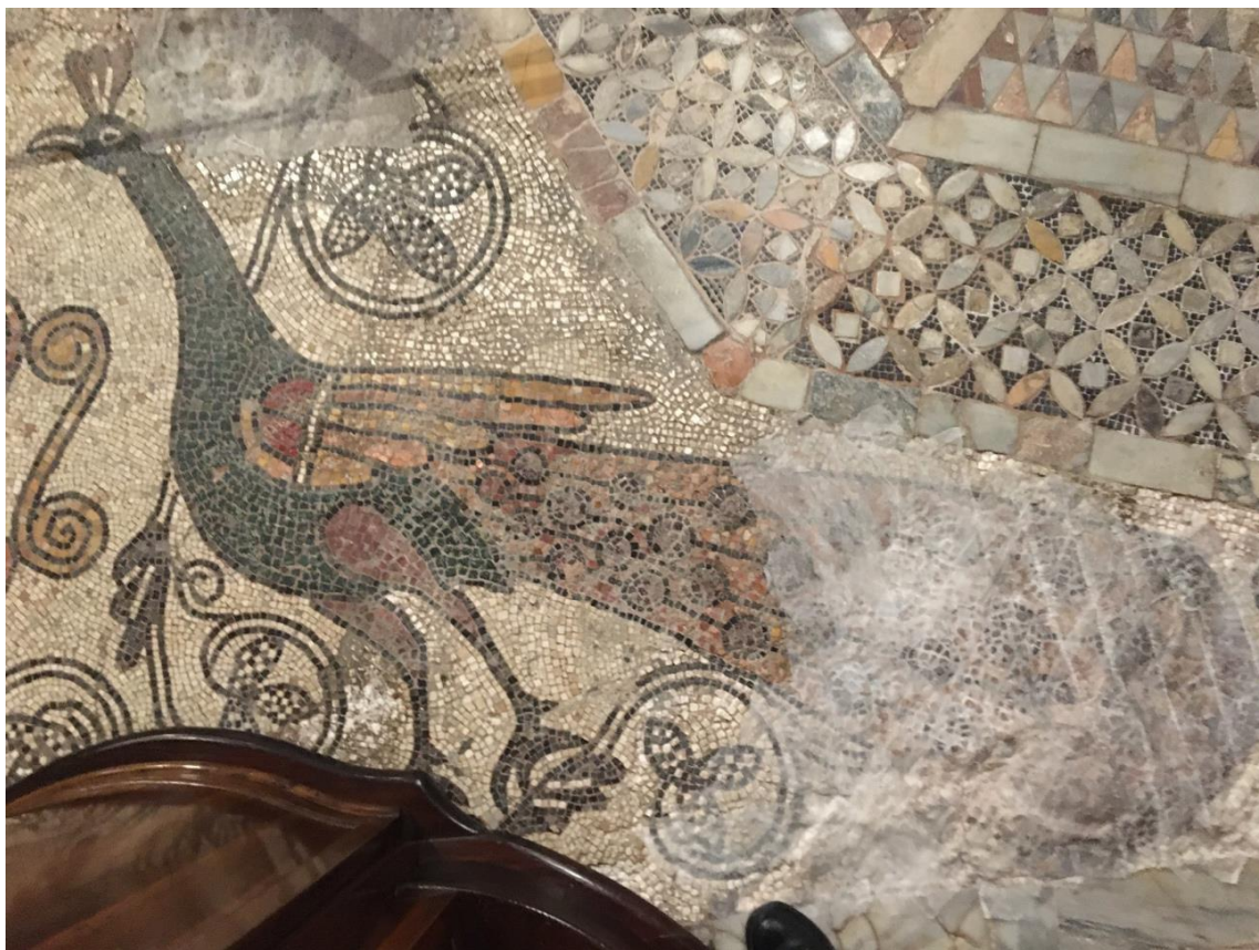
Basilica di San Marco. Parts of the floor's surface with the mosaics have been raised; the mosaics are secured by a fleece paper (Bernhard Furrer)
