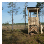
View of newly built bird tower. ( Länsstyrelsen Västernorrland, 02-10-2013 )
