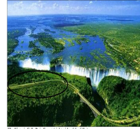
The Victoria Falls Suspension Bridge with a view of the falls
